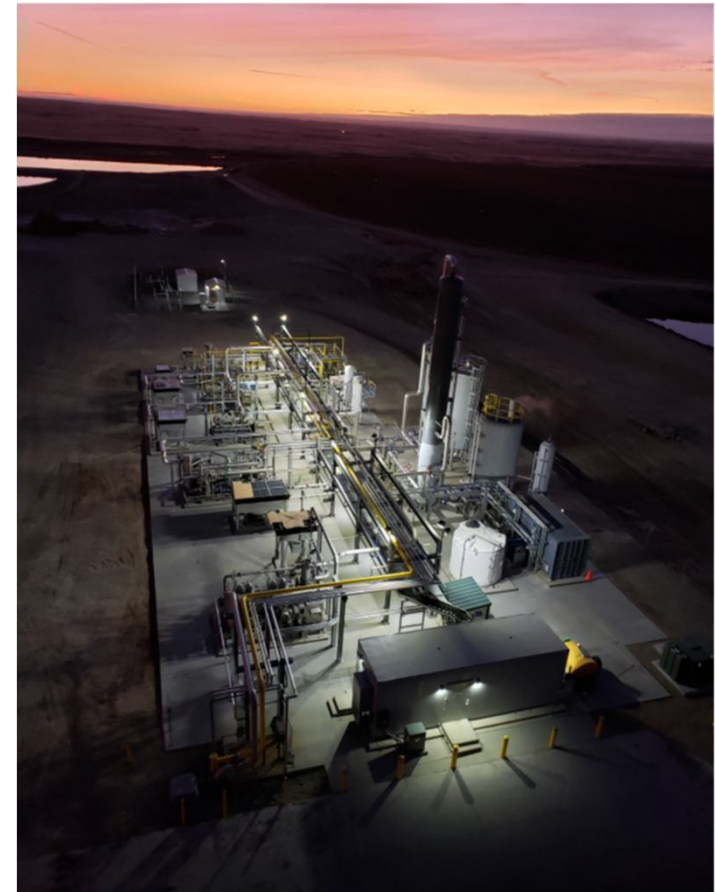
Regenis constructed/operated facility near Jerome Idaho—Dairy Manure 1,200 SCFM raw biogas
