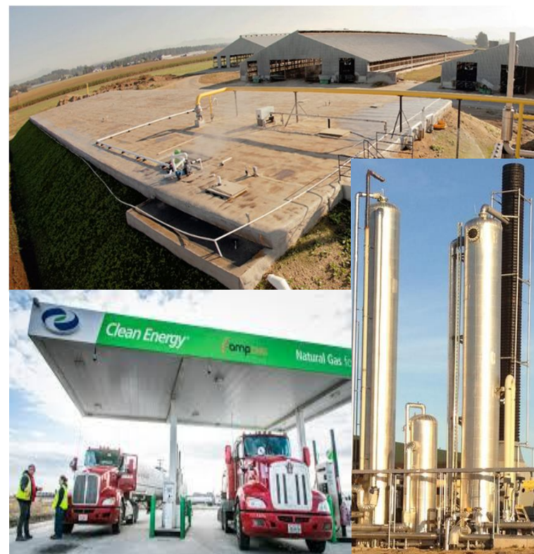
(a) Dairy manure anaerobic digester (Edaleen Dairy, WA); (b) biogas scrubbing (Fair Oaks Dairy, IN); (c) Milk truck fueling with RNG (Fair Oaks IN)
